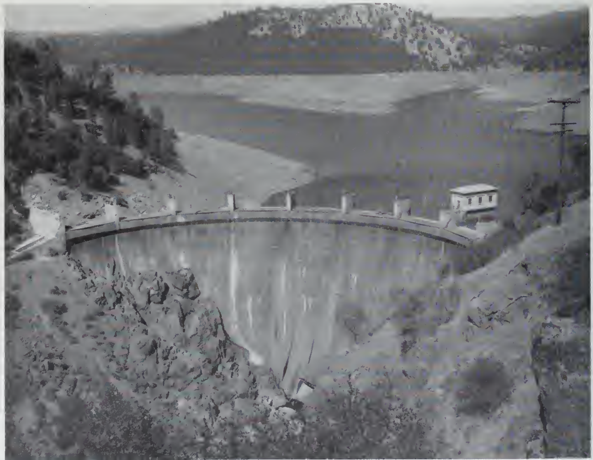
Melones Dam on Stanislaus River, Nearly Empty
